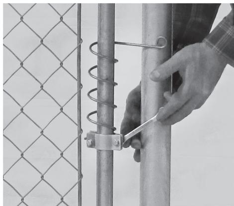
**8.** Adjust spring tension and tighten bolts.
