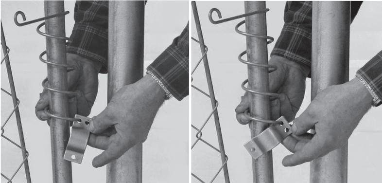
**4.** Insert spring into top right hole of front clamp piece and rotate into place.
