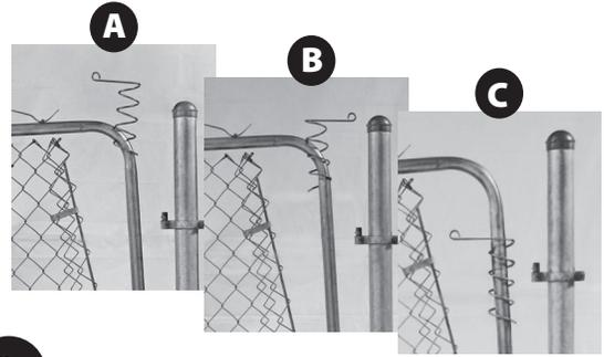
**3.** Rotate Gate Shut spring onto top corner of gate.
