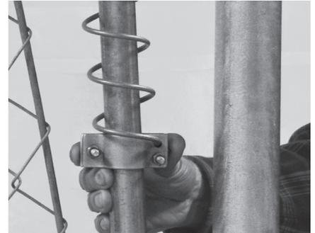
**5.** Place back piece of clamp and install bolts finger tight.
